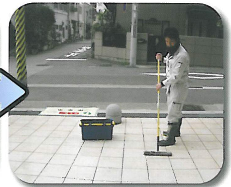
●二次液剤塗布作業●
